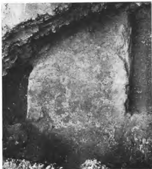
Fig. 105 — S. Lorenzo f.l.m. Basilica maior , dig 6, facade wall, looking north (Photo: Sansaini).
